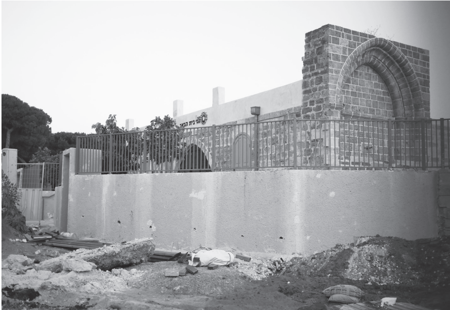
Well House in 16 Pinkhas Lavon St. Maya Yavin
